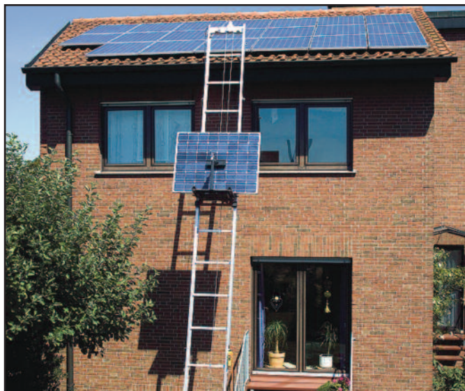
Mathand 150 Solar inclined to building without bend section (compulsory safety rails have been removed for this promotional image)
